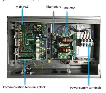
Figure 5-1.4: 14-20HP bottom layer of electric control box
