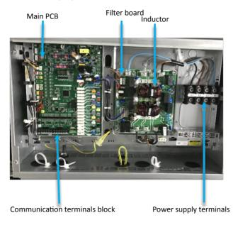
Figure 5-1.2: 8-12HP bottom layer of electric control box
